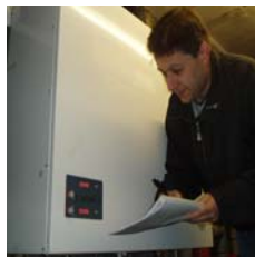
Checking new boiler readings at Cedar Manor
